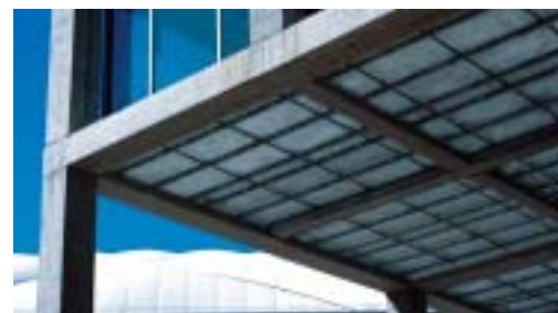
Soffit application to insulate occupied space above
