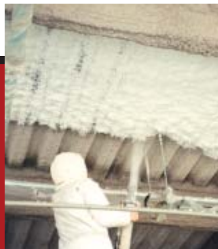
Non-combustible Monoglass applied over fireproofing; University of California
