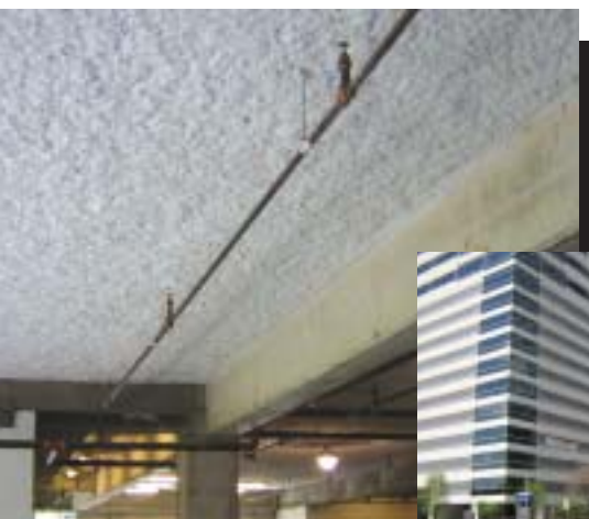
Acoustic Spray-On Application
