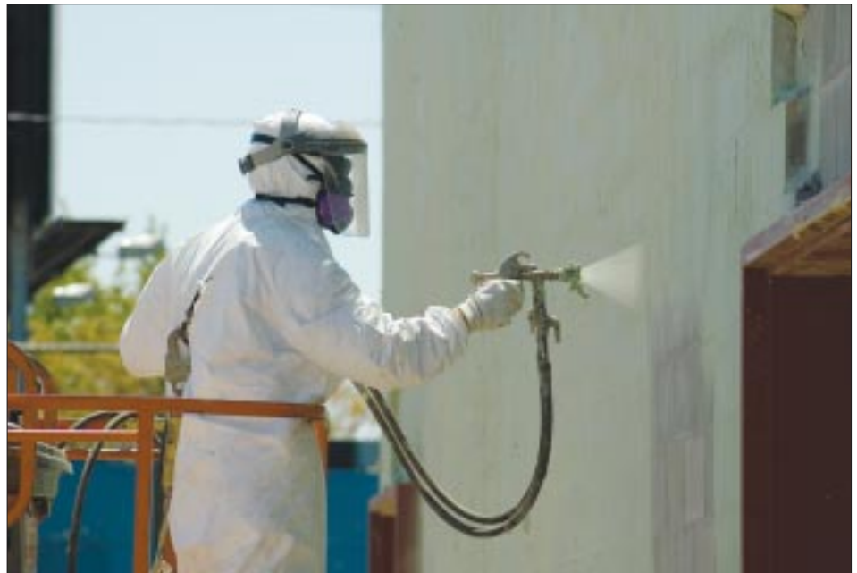
Spray applied Perm-A-Barrier ® Liquid, an air and vapor barrier
