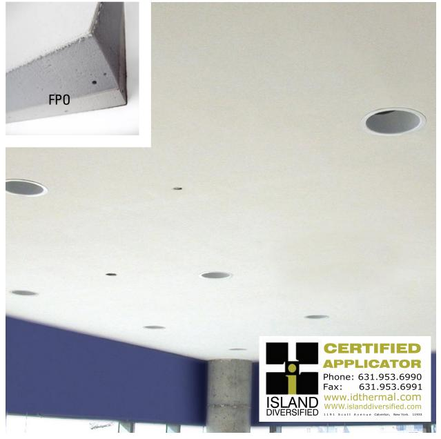
Class 1 fire-rated, SONEX<sup>®</sup> AFS (Acoustical Finish System) offers excellent acoustical control with an attractive monolithic, slightly textured finish to walls and ceilings. PHONSTOP<sup>®</sup> PA85 Plaster is applied in two thin layers over a fiberglass mesh pre-affixed to pinta's willtec<sup>®</sup> foam panels—providing a finished look similar to porous drywall. Color can be applied using a non-bridging coating to compliment nearly any décor.
